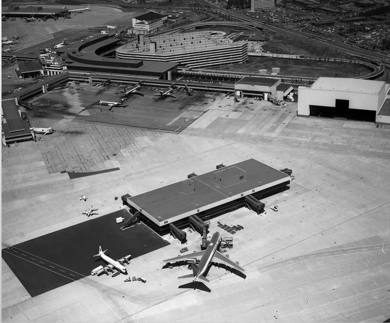
Single Aircraft at South Satellite in 1971 – HVAC System Installed
